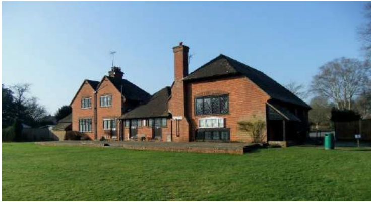
Rear of Village Club with adjoining steward's accommodation
