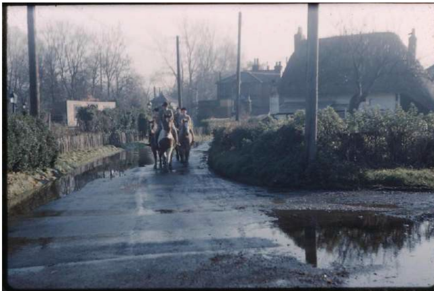
Photo 1 – Flooding at north end of Village Street, outside Yew Tree Cottage, 1960
