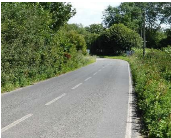
Road from Upper Clatford entering the village
