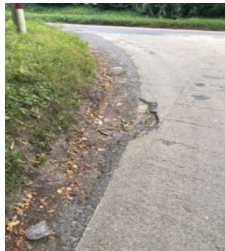
Junction of Church Lane with the A 3057
