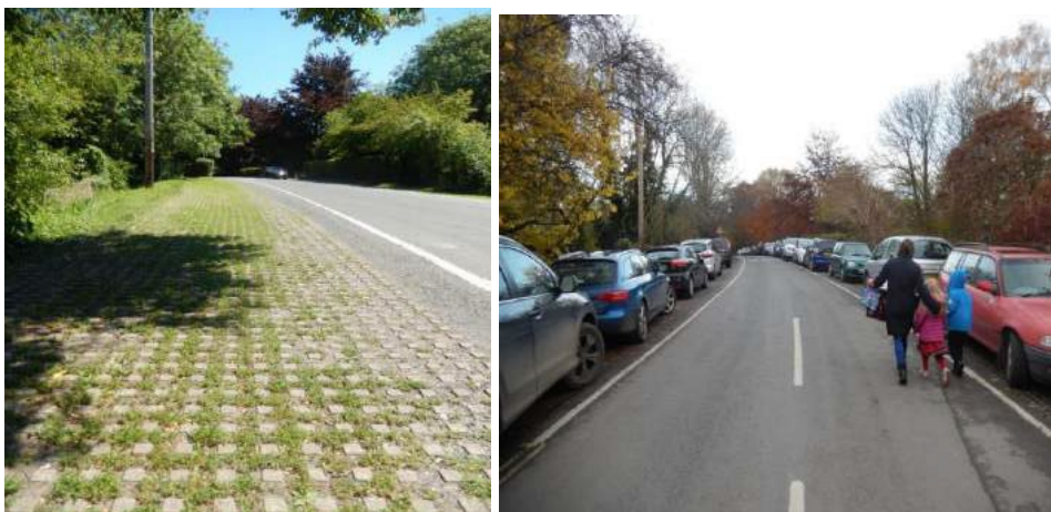
Grasscrete laid either side of the road created additional parking.
