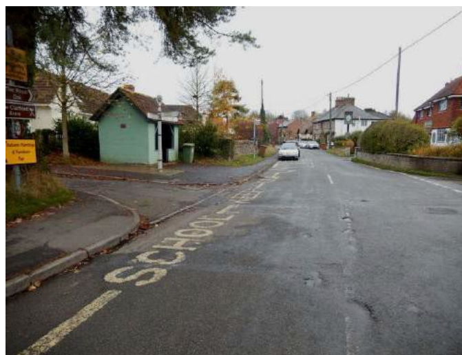
Unclear markings outside the School - Longstock Road
